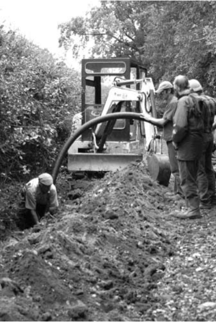
Vital work laying a pipe to help drain a bridleway. Steve Jones is the man in the ditch.
